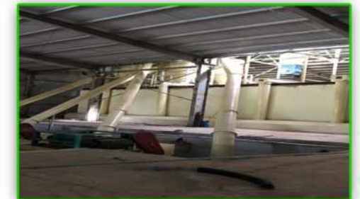
Hydraulic material push warehouse
