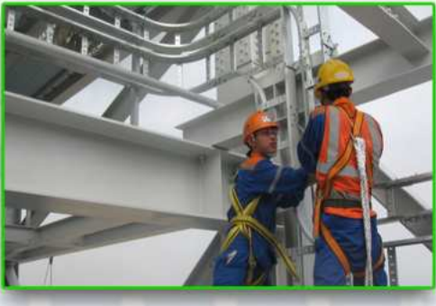
Electrical system construction
