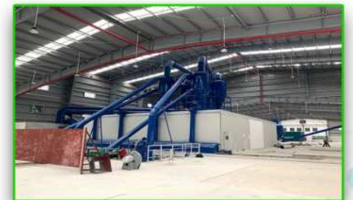
Hydraulic material push warehouse
