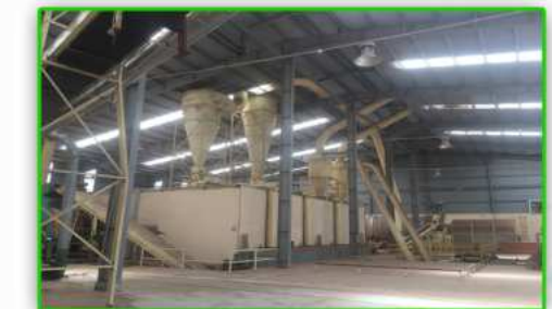
Hydraulic material push warehouse
