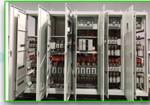
Assembling electrical cabinets
